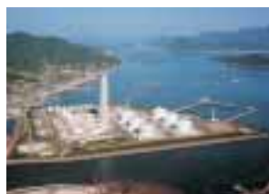
Yanai Thermal Power Station (LNG)
