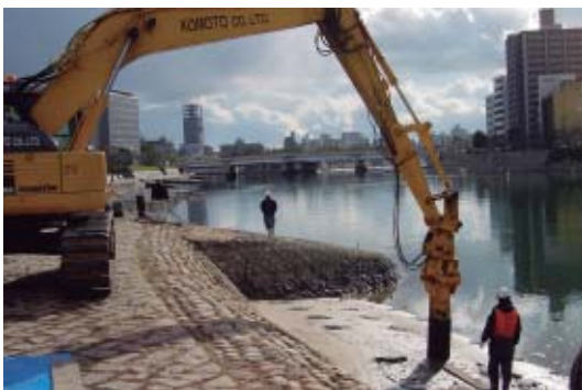
Osmotic column, made from coal ash products, for improving soil water retention
