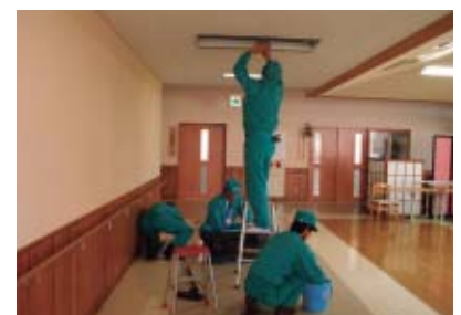
Cleaning electrical equipment at a social welfare facility
