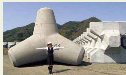
Large breakwater blocks (20–80t) at a nuclear power station are made with coal ash produced at coal-fired thermal generating stations.
