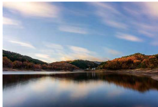
Onbara Dam (Kagaminno-cho, Okayama Prefecture), the oldest buttress dam for power generation in Japan, surrounded by lush forests of white birch, larch, and other trees
