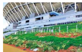
Artificial soil was used in the slopes on the northeast side of a football stadium in Hiroshima (Light Sand)
