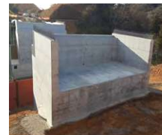
Concrete admixture used in a pedestrian bridge over the Oda Shizuma Road in Shimane Pref. (Eco-powder)
