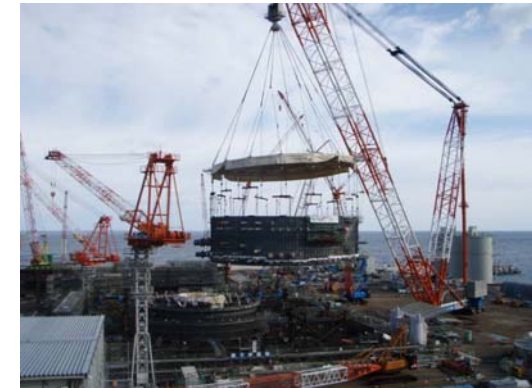
Overview of the Shimane nuclear Unit No3 construction site (September, 2008)
