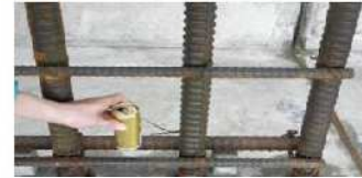
Reinforcing bars of up to 51 mm in diameter are used.
