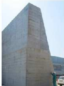
Breakwater following concrete placement
