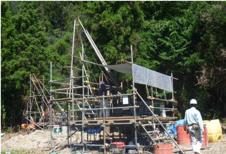
Drilling survey in progress
