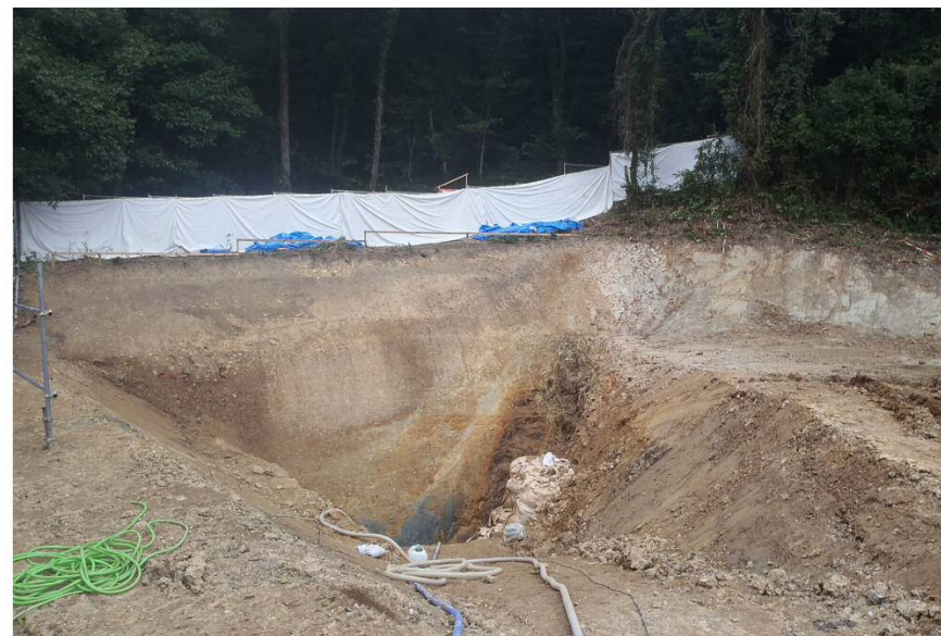
Trench survey in progress
