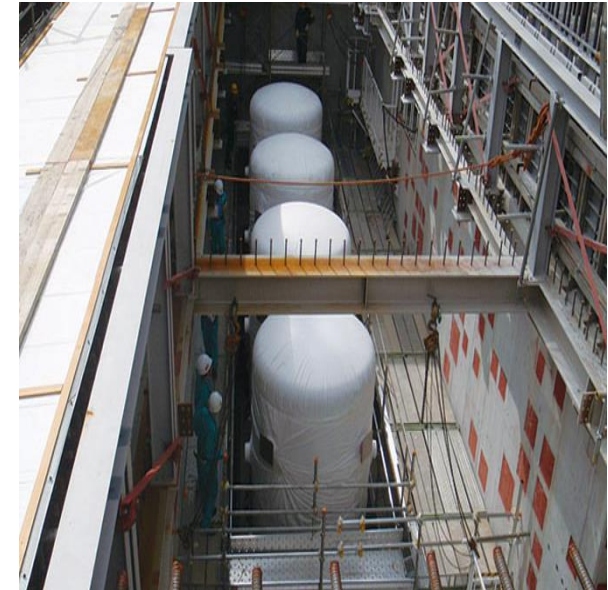
Filtered Vent Equipment
