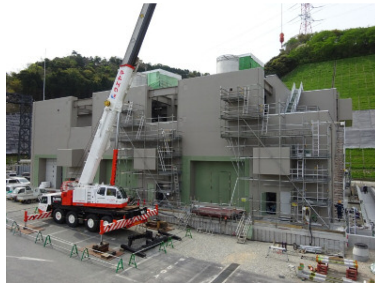
Installation of a gas turbine generator (As of April 2017)
