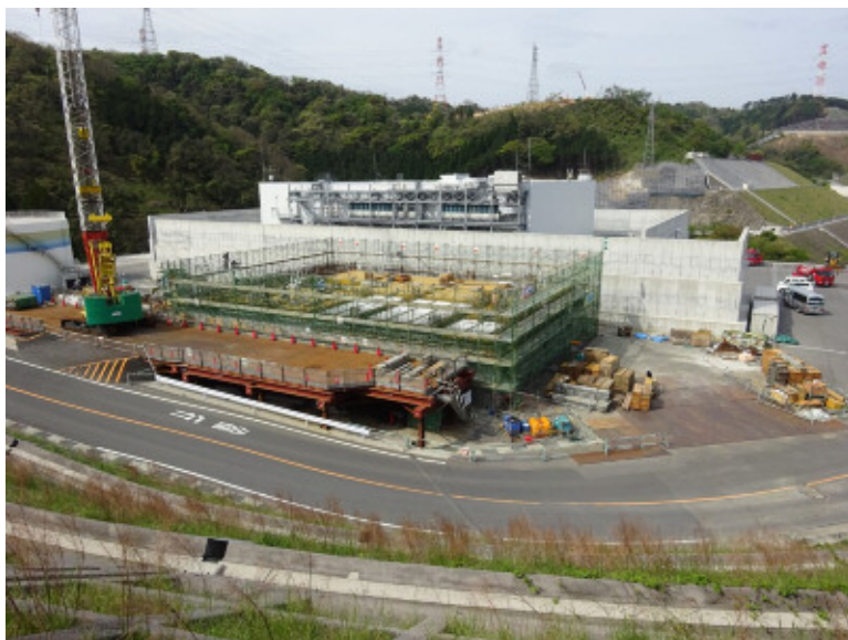
Installation of an emergency response facility (As of April 2017)
