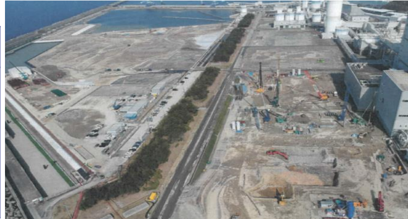
[ State of Construction ] (As of February 2019)
