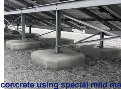
A concrete using special mild material (CO 2 -SUICOM)
