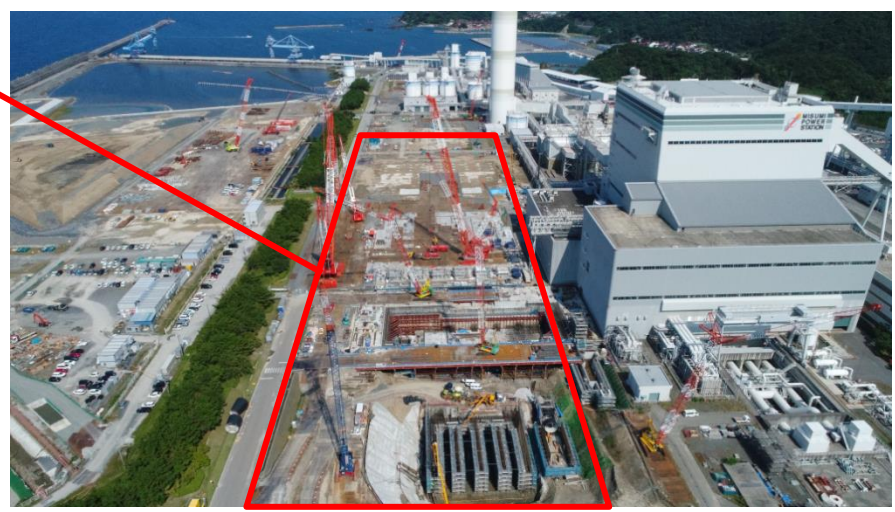
[State of Construction] (As of August 2019)
