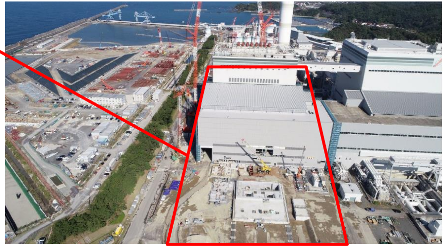
[State of Construction] (As of October 2020)
