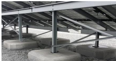
A concrete using special mild material ( CO 2 -SUICOM )
