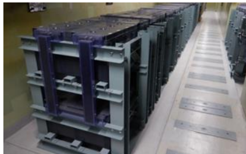
Improvement of storage batteries to ensure DC power supply
