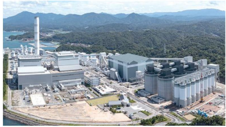
View of the Misumi Power Station
