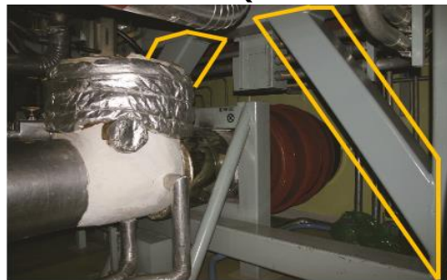
Equipment/piping/other seismic reinforcement work (Unit 2)
