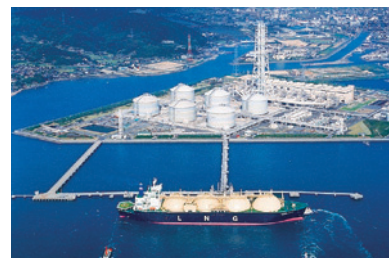
LNG vessel alongside Yanai Power Station
