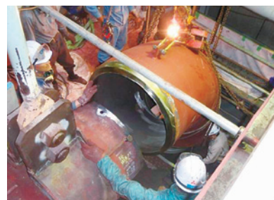
Replacing boiler tubing at Misumi Power Station
