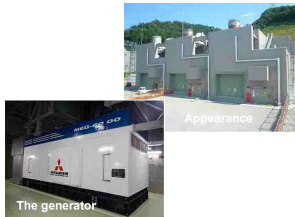
Installation of a gas turbine generator (As of July 2019)
