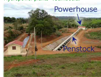
Consulting for Development of Small-scale Hydropower plants (Cambodia)
