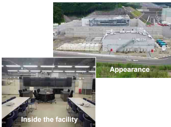
Installation of an emergency response facility (As of July 2019)
