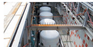
Installation of filtered venting systems
