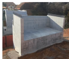
Concrete admixture used in a pedestrian bridge over the Oda Shizuma Road (Eco-powder)
