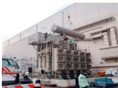
Work to remove main transformers and indoor transformers
