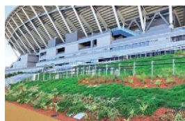
Artificial soil was used in the slopes on the northeast side of a football stadium in Hiroshima (Light Sand)
