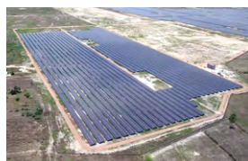
Power station exterior (drone aerial photo)
